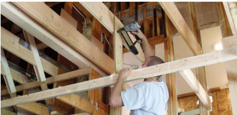
**Figure 3.** When the truss modifications were complete, the crew cut out the original bottom chords to leave a recessed space for the barrel vault (top). A 2x4 around the perimeter (above), positioned  $\frac{3}{4}$  inch above the surrounding soffit, would accommodate a shelf for LED uplighting.
