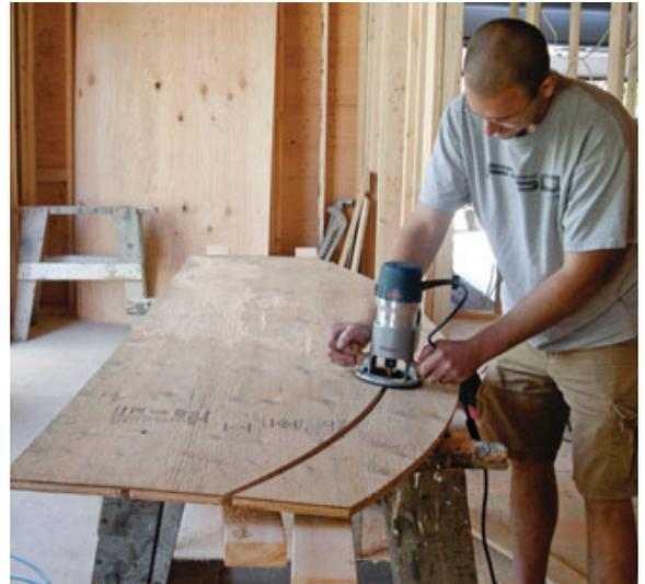
**Figure 4.** Working on the deck, a carpenter routs arcs in a sheet of plywood, but without cutting through to the subfloor (above). The arcs are completed on the bench with a pilot bit (above right), then laminated with glue and staples to form ribs long enough to span the vault (right).
