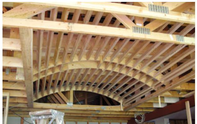
**Figure 5.** The vault framing was too heavy to install as a prebuilt unit, so it was assembled in place (left). Ductwork for a commercial range hood will run through the opening between the two center ribs (above).
