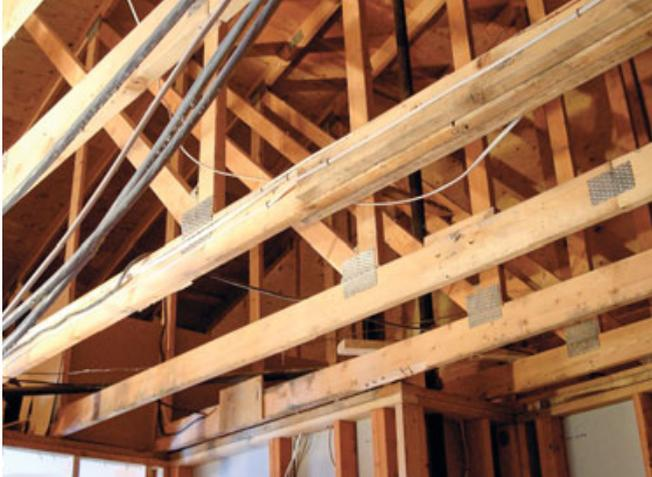
**Figure 2.** After stripping off the ceiling to expose the existing trusses (above), the crew shortened vertical and diagonal webs to install a new 2x10 bottom chord, reinforcing the connections with plywood gussets and staples (right).
